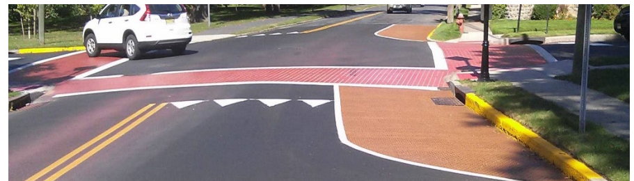
Figure 19. Painted crosswalks and bumpouts.
