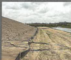
OVERWHELMED SILT FENCE
