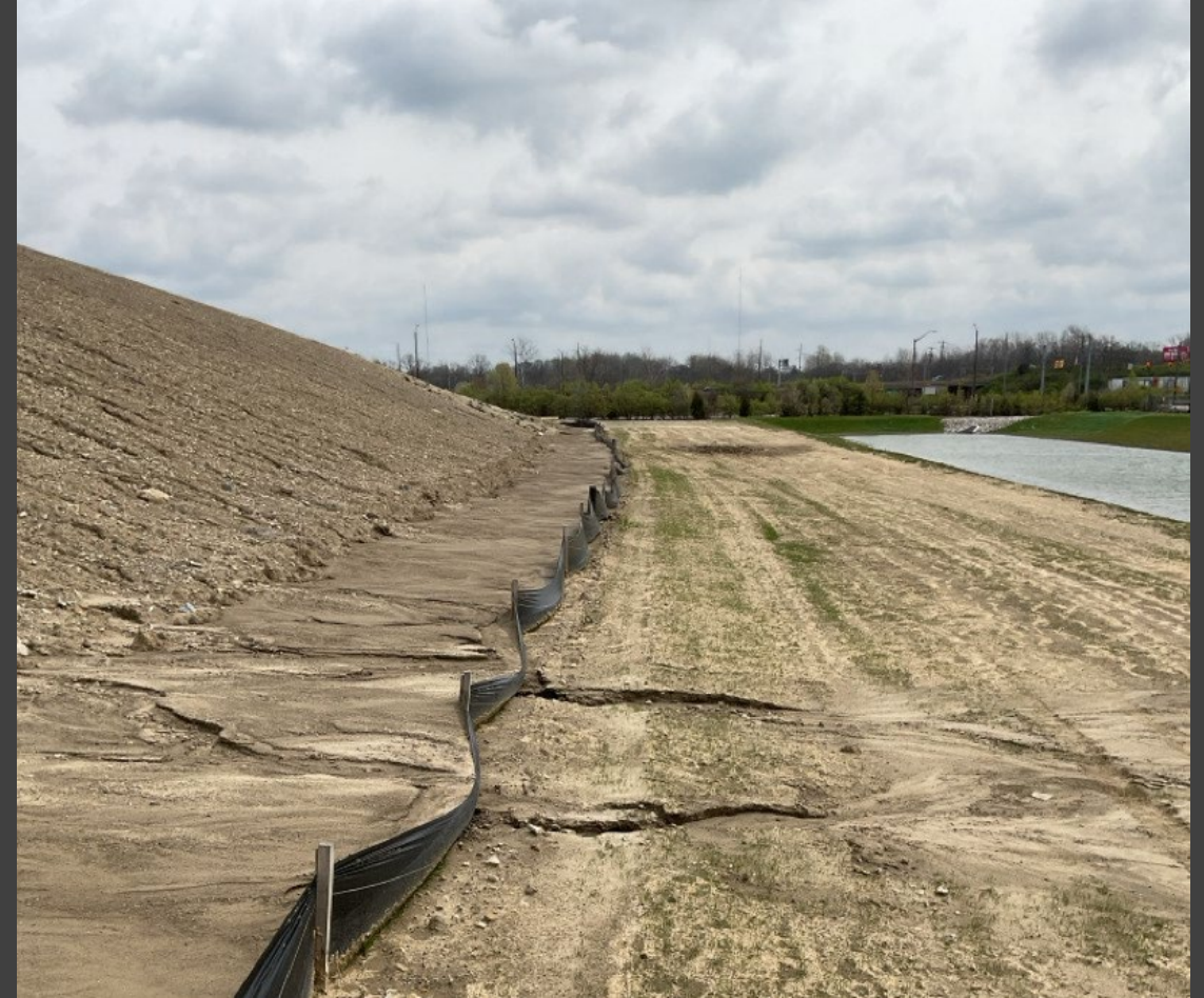
OVERWHELMED SILT FENCE
